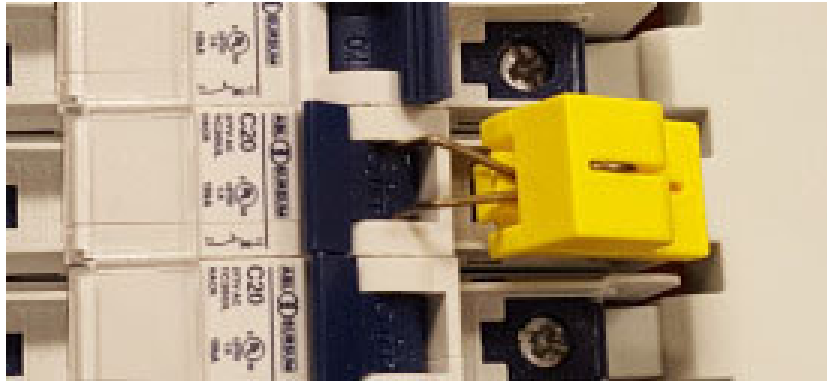
Figure 3.3.1-2 STEP 3: LOCKOUT ATTACHED
